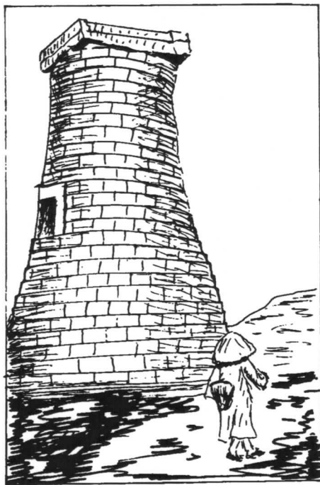
Fig. 109. Bottle-like geometrically stable form of the Star tower
